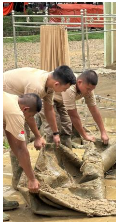
Gambar 2. Rehabilitasi interior mushola pascabanjir.
